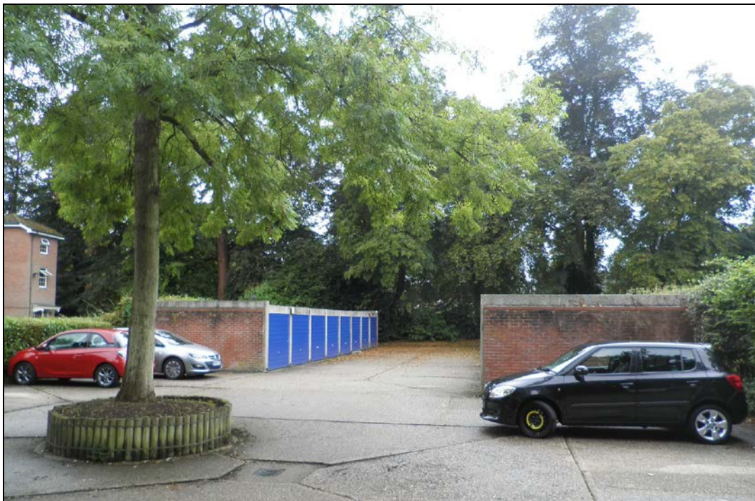
Garage Court/Car Park
