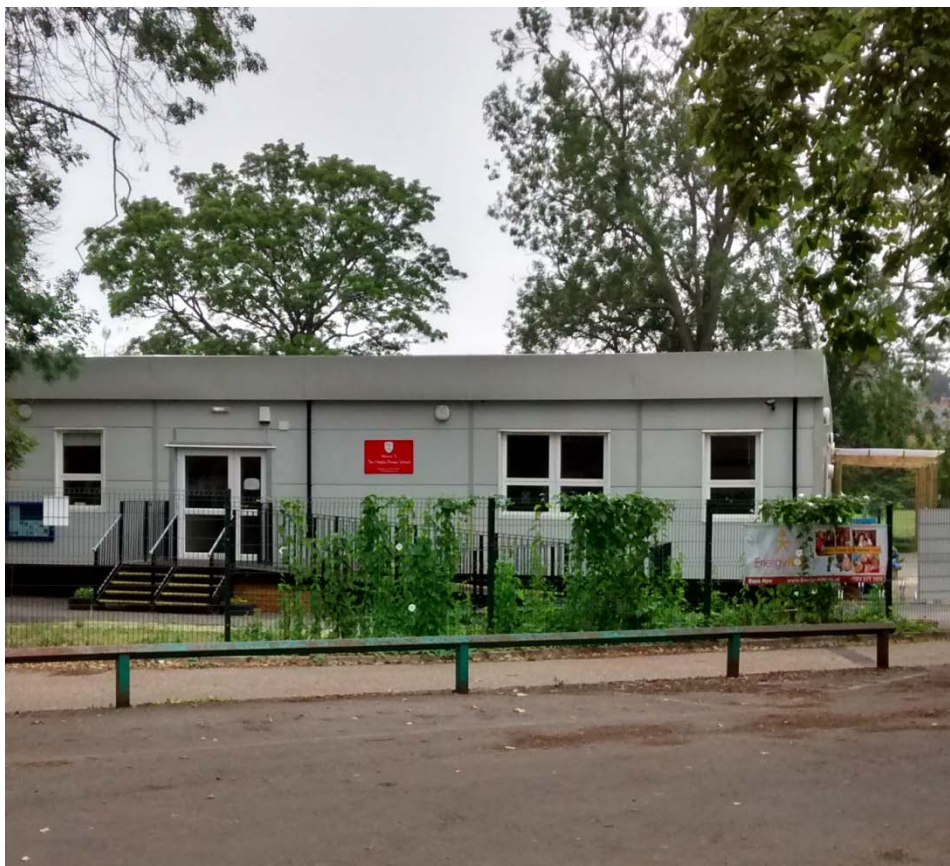
View of existing school from the front (south elevation)
